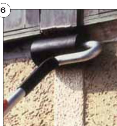
Remove excess caulk, trim ends and terminate with a cap bead of 864NST
