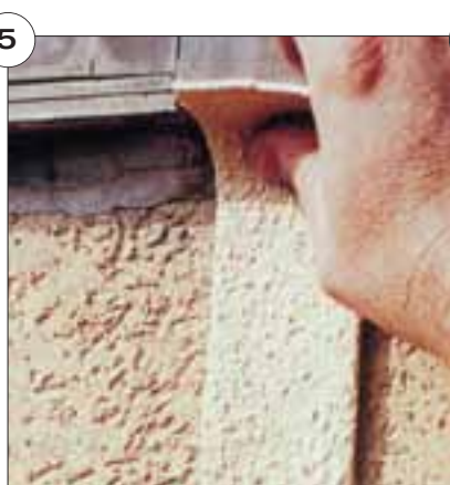
Apply Sil-Span to the prepared joint substrate
