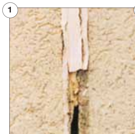
Sealant failure in expansion joint
